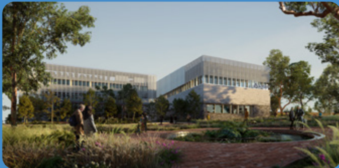
Second Building construction
