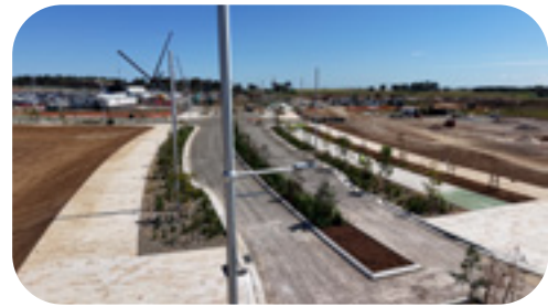
Enabling infrastructure in Bradfield City
